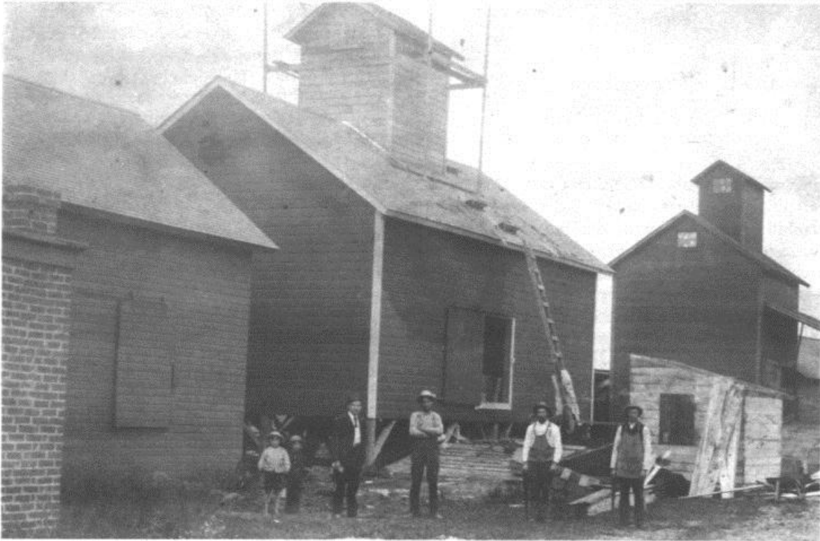
Fred Lyons and crew putting the finishing touches on his new elevator in 1904. The Northern Grain & Seed elevator is on the right.
