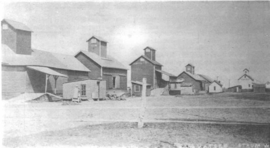
The elevators, taken before 1912. Left to right, T. M. Olson's, Fred Lyon's, Northern Grain & Seed, Cargill. Of those pictured, only the Strum Mills building at far right still stands.
