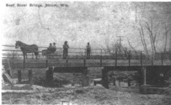
The Beef River Bridge, about 1910.
